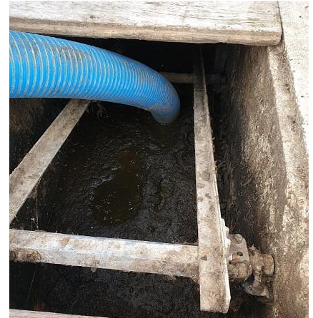
Figure 1- Liquid manure in pit
