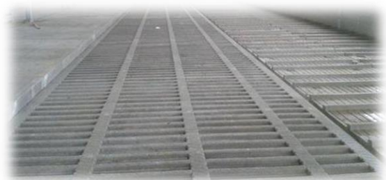
Figure 2- Typical flooring in a Dutch cow shed
